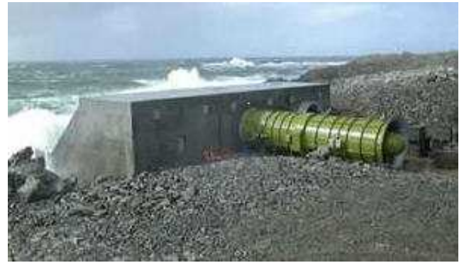
Figure 3: Shore Oscillating Water Column [3]
